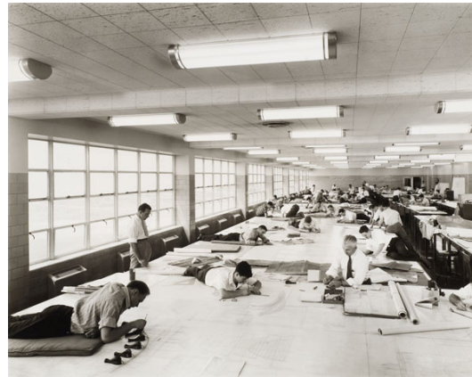
Ford Motor bomber factory, Willow Run, Michigan, by Albert Kahn Associates, view of the drafting room, 1942. Photograph by Hedrich-Blessing. CCA Collection PH2000:0393. Gift of Federico Bucci. © Chicago History Museum, HB-07074-G
