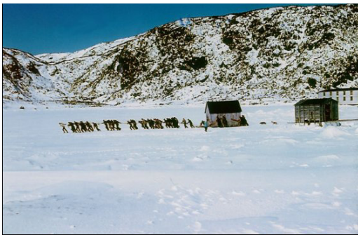
Pulling a structure across the ice to Conche, Newfoundland. Resettlement Collection, Maritime History Archive, Memorial University, PF-317.488
