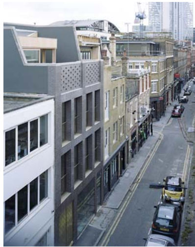
Stephen Taylor, architect. David Grandorge, photographer. House on Charlotte Road, London, 2008. © David Grandorge.
