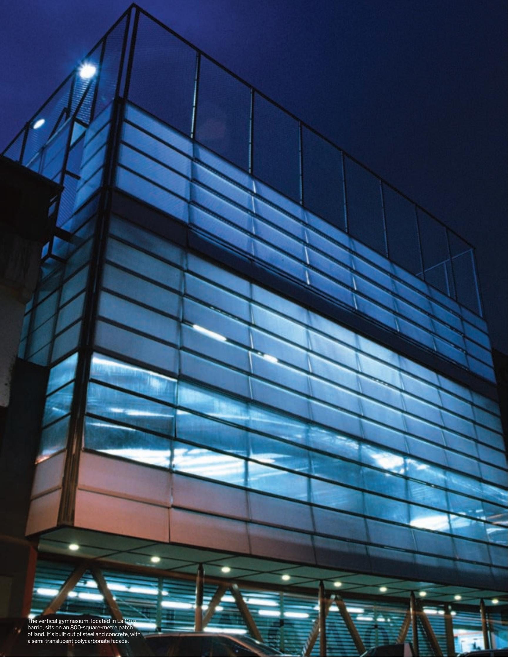
The vertical gymnasium, located in La Cruz barrio, sits on an 800-square-metre patch of land. It's built out of steel and concrete, with a semi-translucent polycarbonate facade.
